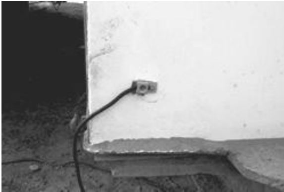
Note single metal-to-metal connection
