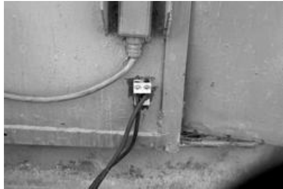
Note double metal-to-metal connection
